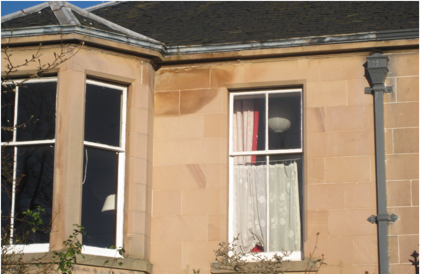
Figure 2: Damp penetration (image © Historic Environment Scotland)
