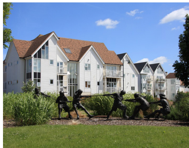
Figure 22: Apartment block, Kings Hill (© LPT)
