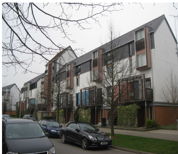
Figure 6: Housing on 'The Chase'
