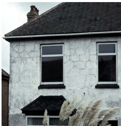
Figure 3: Photographs of two different properties exhibiting characteristic mundic damage
