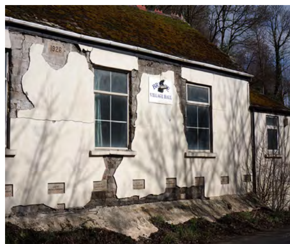
Figure 3: Photographs of two different properties exhibiting characteristic mundic damage
