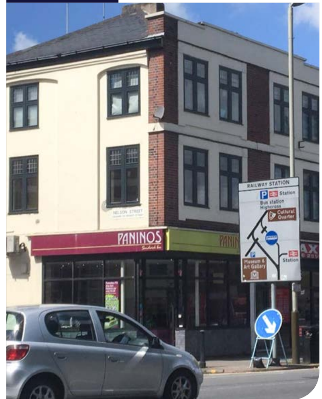
The appearance of 53a London Road on the site visit
