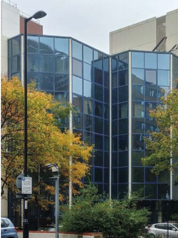
The appearance of 5 Sydenham Road on the site visit
