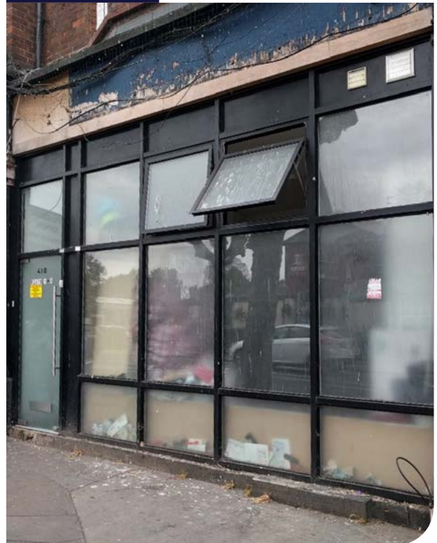
Figure 37 The appearance of 410 Brighton Road on the site visit
