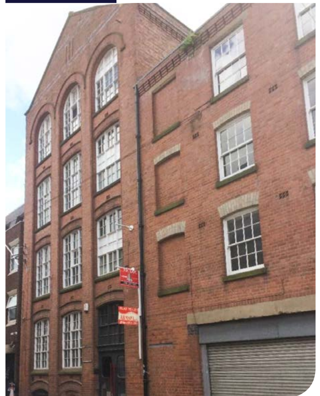
The appearance of Lionel House on the site visit
