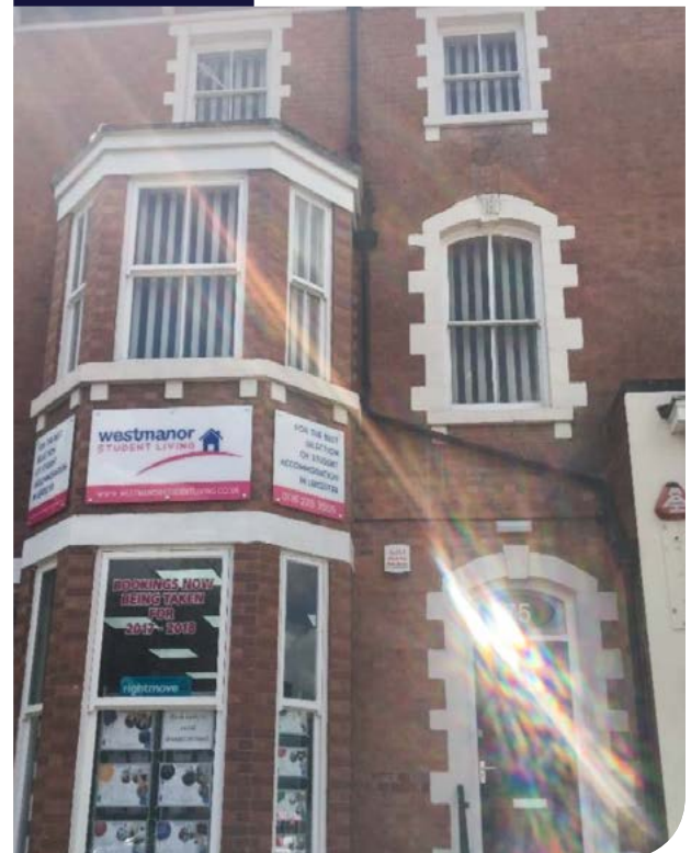
The appearance of 75 London Road on the site visit
