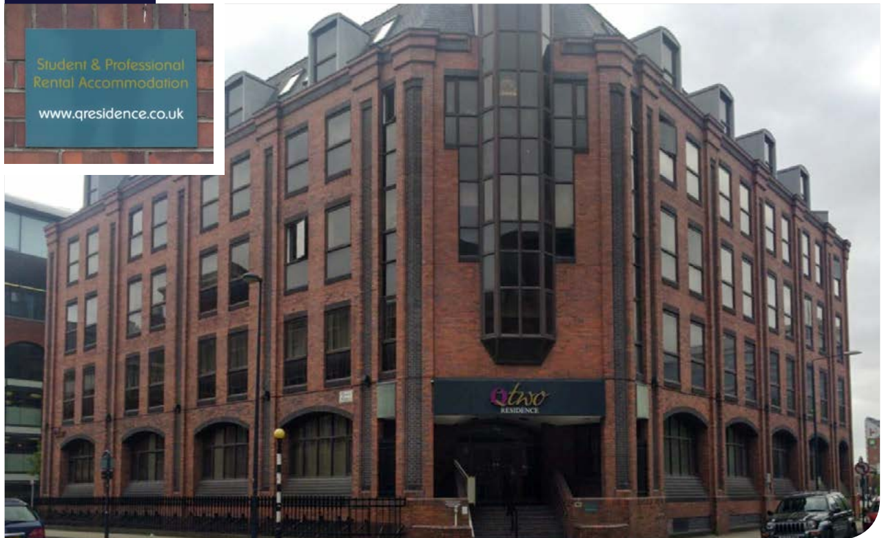
Figure 45+46 The appearance of 25 Queen Street on the site visit and signage at entrance
