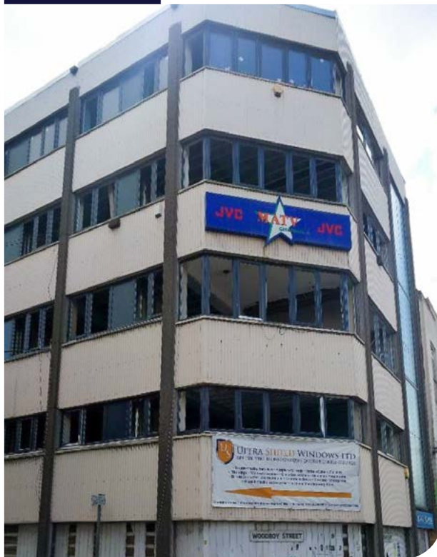
The appearance of MPK House on the site visit, with apparently stalled conversion
