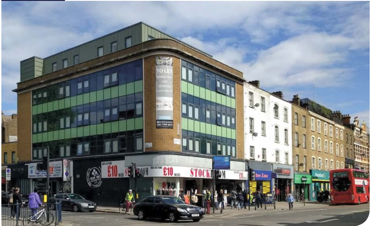
Figure 14 The appearance of Merlin House on the site visit
