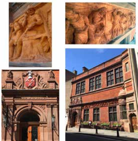
Cutlers Hall, City of London. After conservation City Heritage Award for the Conservation & Refurbishments of the Facade, including Terracotta Frieze & Coat of Arms
