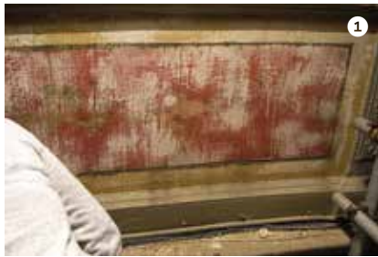
1 Upper circle box painted panelled front behind the 1832 facade
