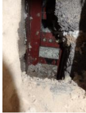
Opening up the cavity showed the base of the steel stanchion to be sound in the North corner of the building
