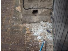
Opening up the cavity showed the base of the steel stanchion to be sound in the North corner of the building
